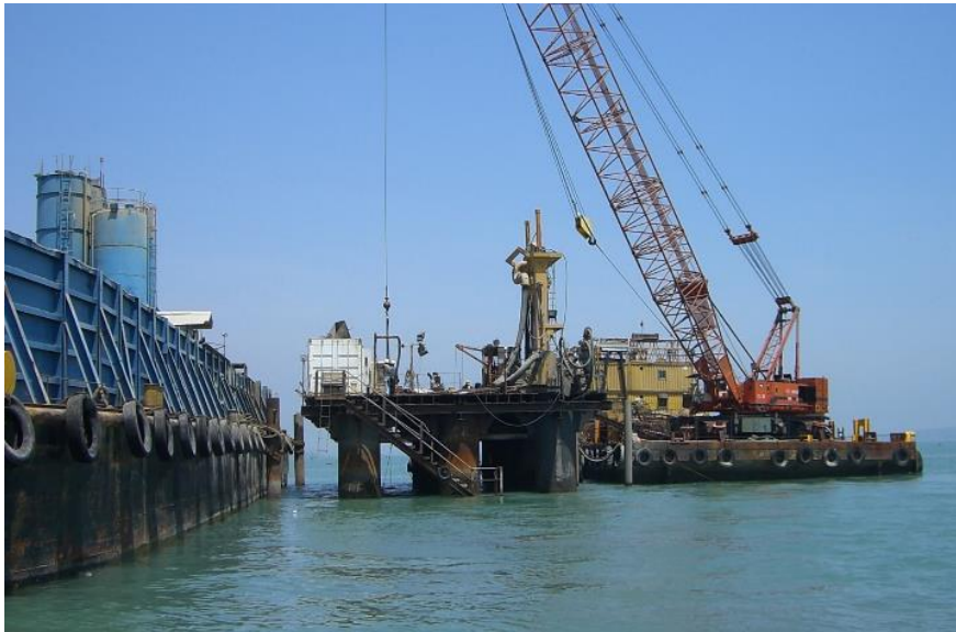
Approach Bridge Suramadu (Drilling for Borep Pile and Concreting with Tremie)
