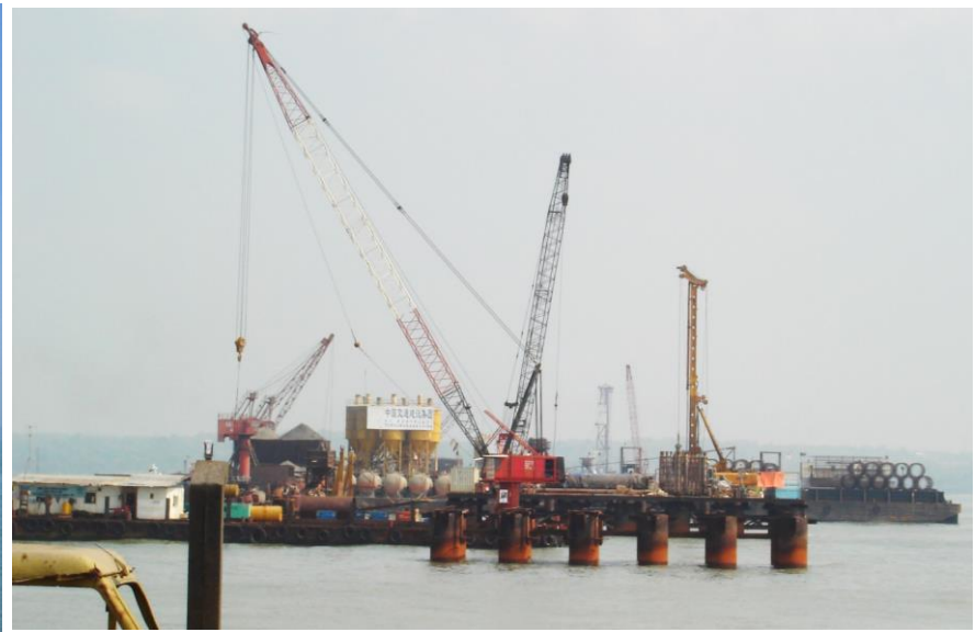
Approach Bridge Suramadu (Drilling for Borep Pile and Concreting with Tremie)
