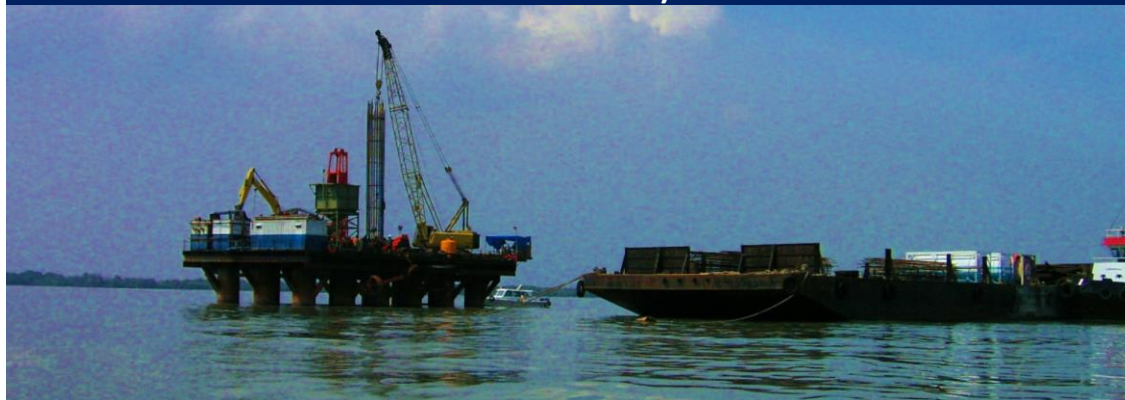
Approach Bridge Suramadu (Drilling for Borep Pile and Concreting with Tremie)
